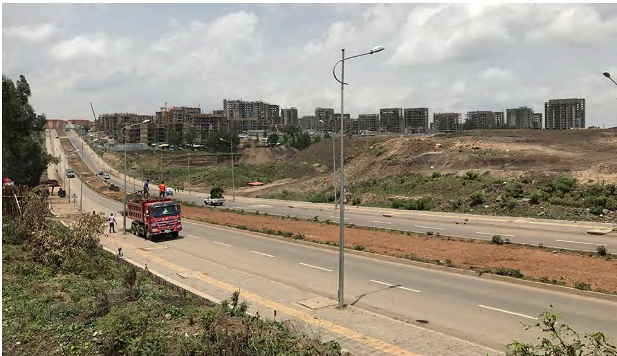
New settlement under construction outside Addis Ababa, Ethiopia (Marcinkoski, 2017)
